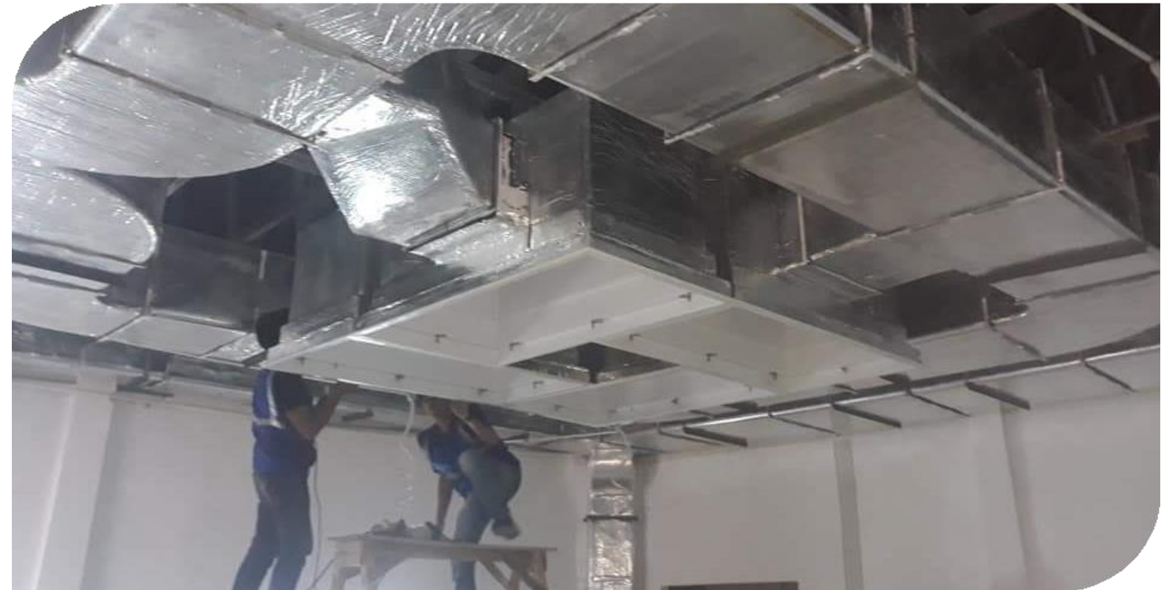
Installation VAC Operating Room – RSPP Jakarta
