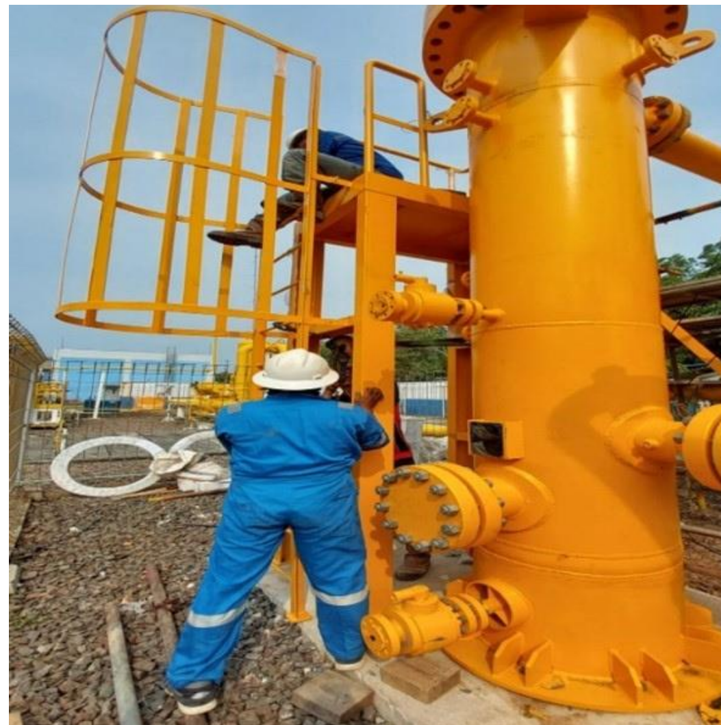
Installation and Commissioning Project Filter Coalescing Vessel at PLTGU Cilegon
