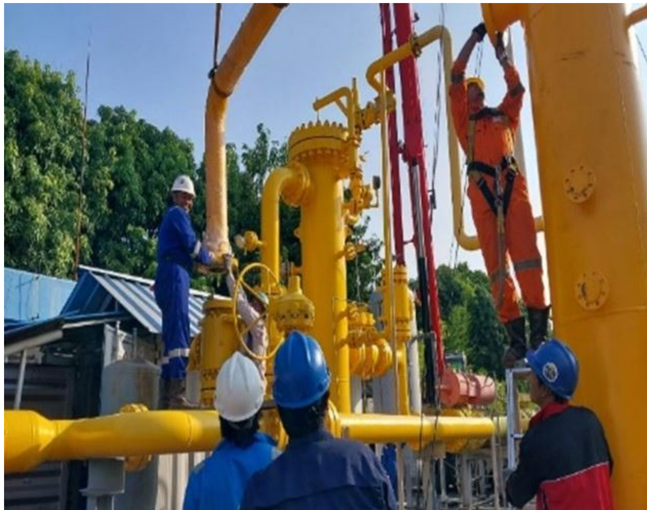
Installation and Commissioning Project Filter Coalescing Vessel at PLTGU Cilegon
